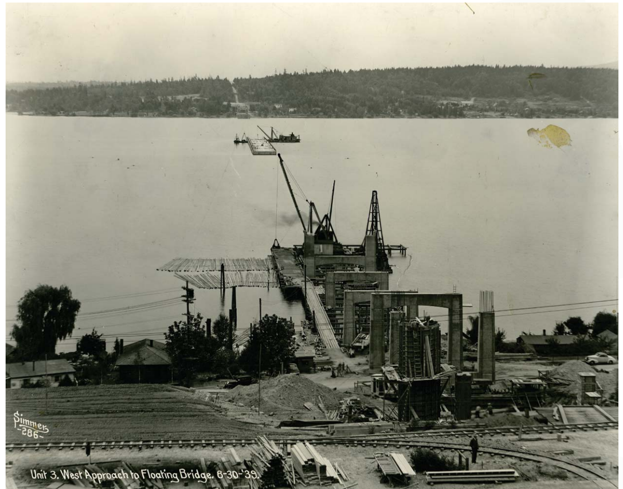
Construction of Lake Washington Floating Bridge, 1939. Courtesy of AAA
